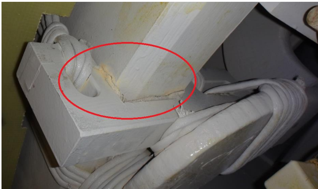
Figure 4 – Loose blocking near 11:00 Jumper Connection in 2015
