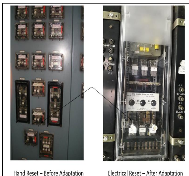
Figure 6. Adaptation of Relays for Remote Reset
