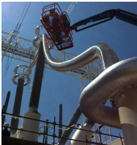
Fig. 5: Mounting of corona shielding and PD free HV line.
