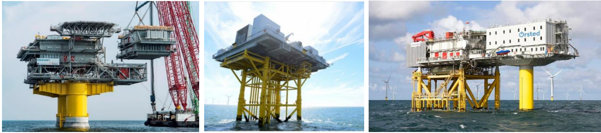
a) Modular topside add-on (Kriegers Flak, Denmark) b) Shared support structure (Humber, UK) c) Adjacent platforms (Horns Rev 2, DK)
