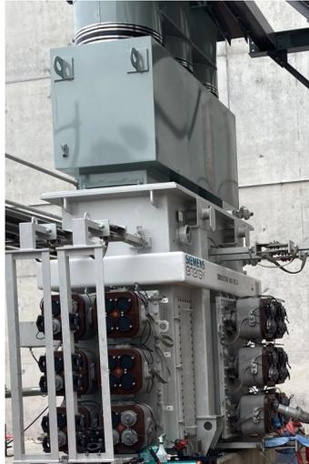
Figure 3- External connection box to connect the single phase transformers to bank configuration
