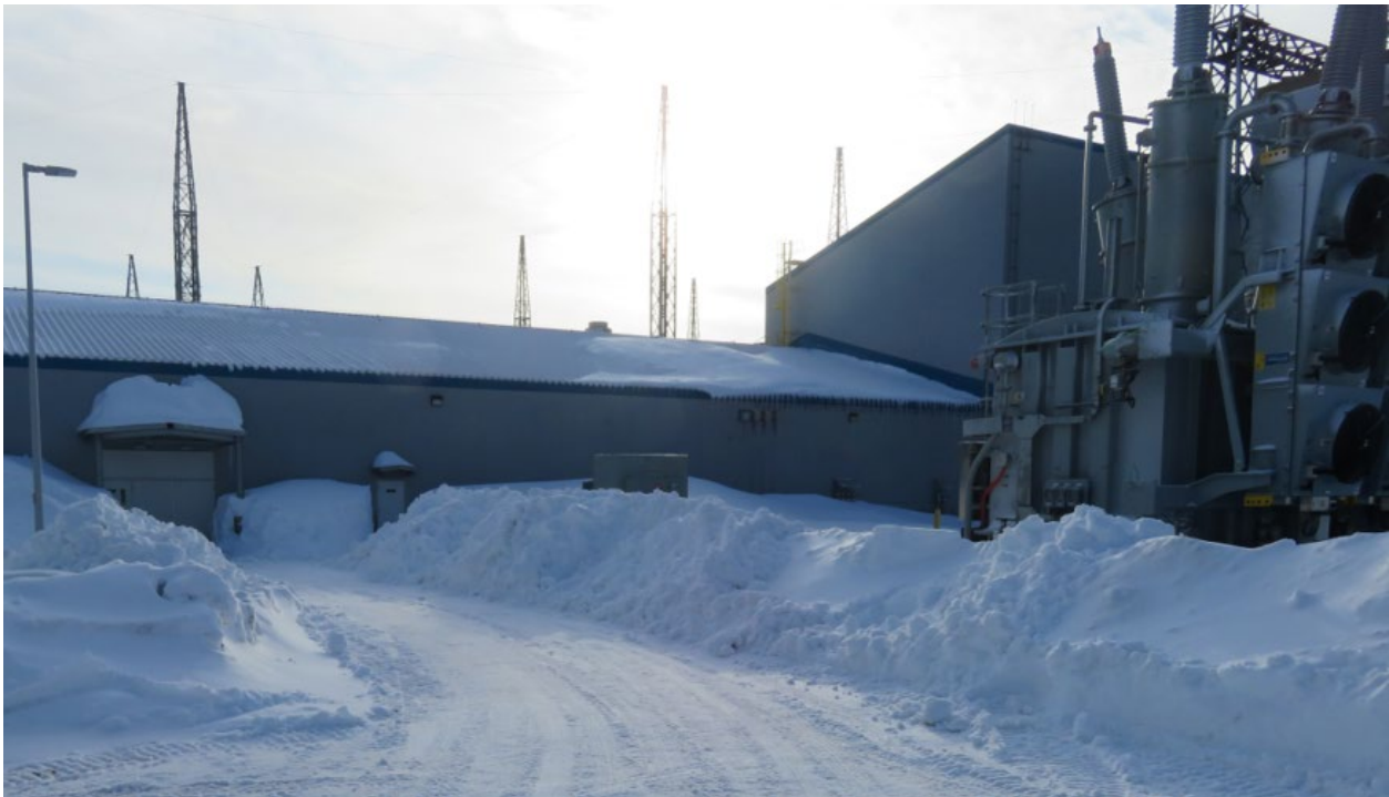
Figure #2 – Snow Accumulation near Control building entrance
