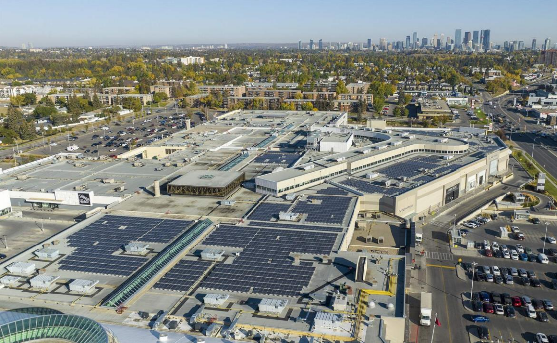
Aerial View of CF Chinook Center Solar Installation
