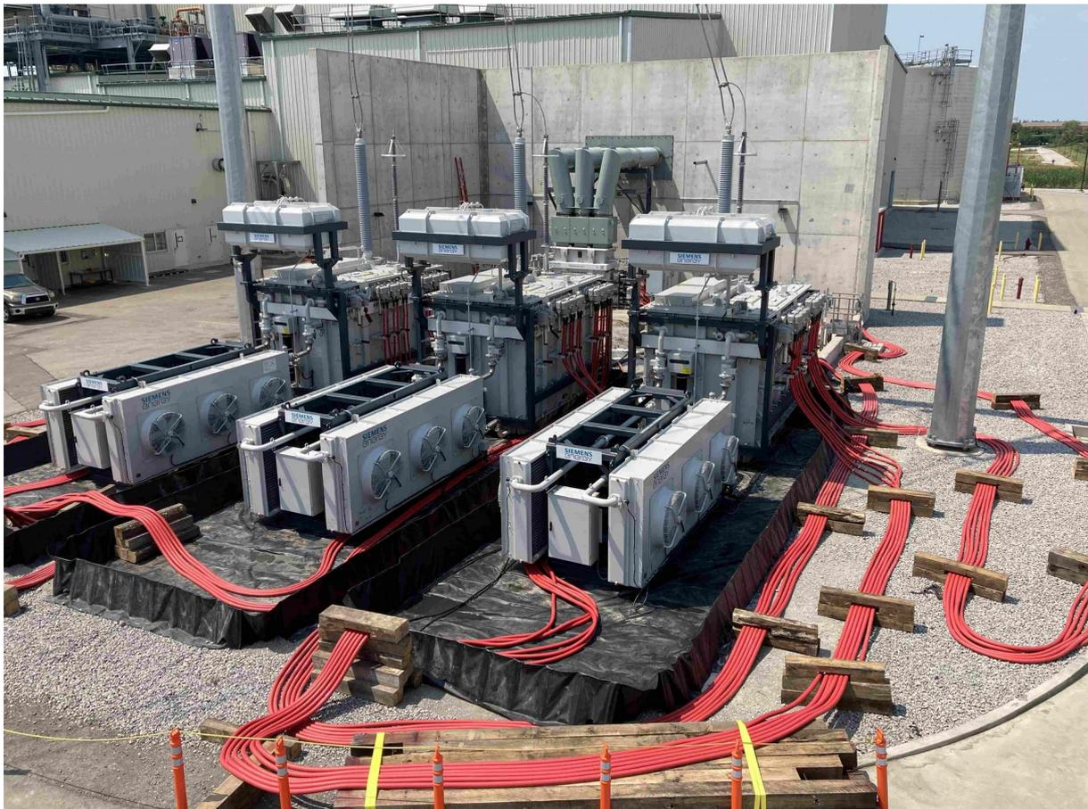
Figure 5 – 250 MVA bank – 345 kV Pretact™ Resilience Generator Step-Up Transformers
