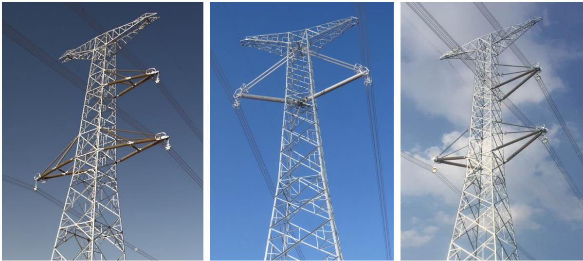
Figure 1. Composite insulated cross-arms in-service on 750 kV EHVAC (left), \pm 800 kV UHVDC (middle) and 1000 kV UHVAC (right) transmission lines.
