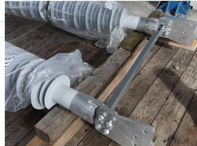
Connection of insulated cross-arm with tower
